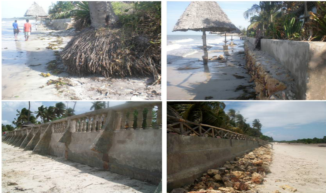
Figure 8: Exposed roots demonstrating beach erosion due to oceanic waves (top left), Sea wall defence at the Millennium Sea Breeze Resort (top right), Sea walls defence at Livingstone Club (bottom left) and Paradise Holiday Resort (bottom right).
